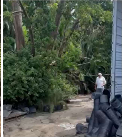
Looking east at site toward access
