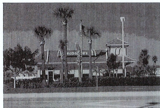
B 1 EXISTING MCDONALDS
