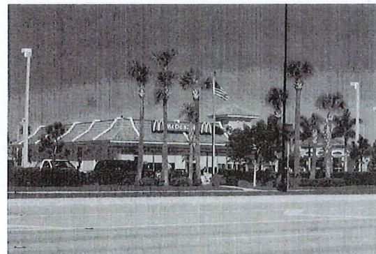
B 2 EXISTING MCDONALDS
