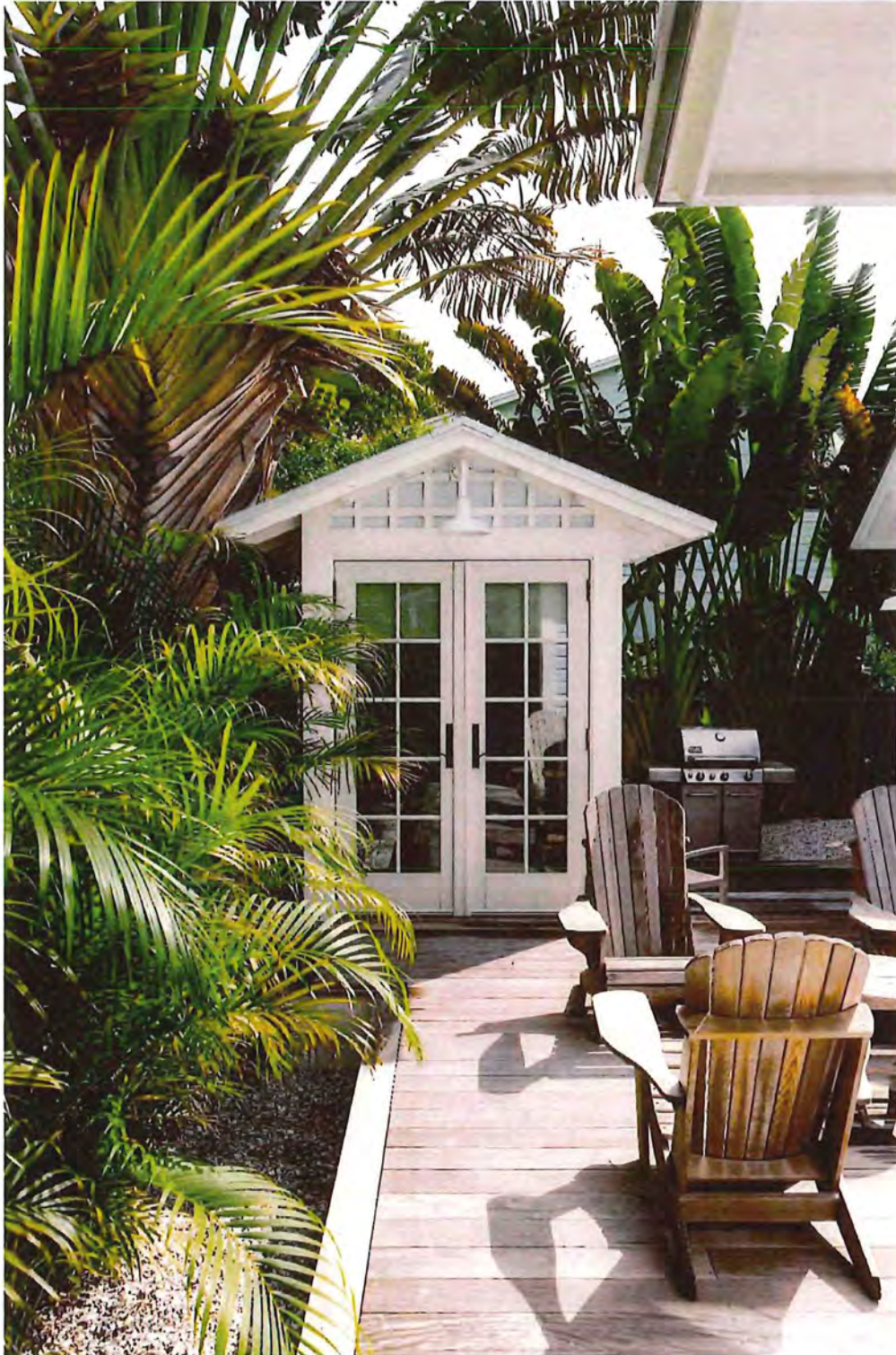
Photo E: West elevation of detached shed taken from northwest corner of wooden deck.
