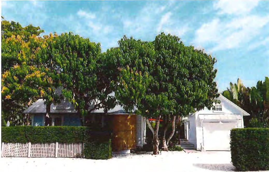
Photo C: South elevation of the main house and garage taken from Waterways Avenue.
