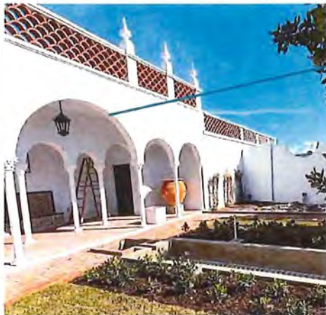
Current photo of the Venetian Pavilion adjoining the unroofed utility courtyard. The new roofed garage will not impact the Venetian Pavilion
