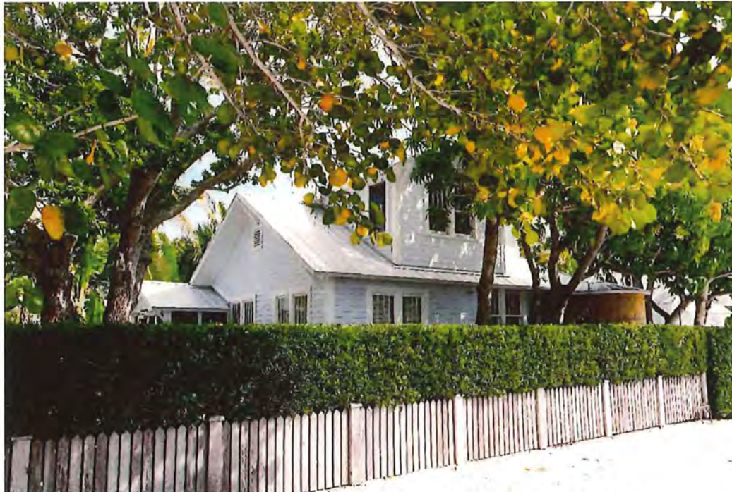
Photo B: Southwest corner of the main house taken from Waterways Avenue.
