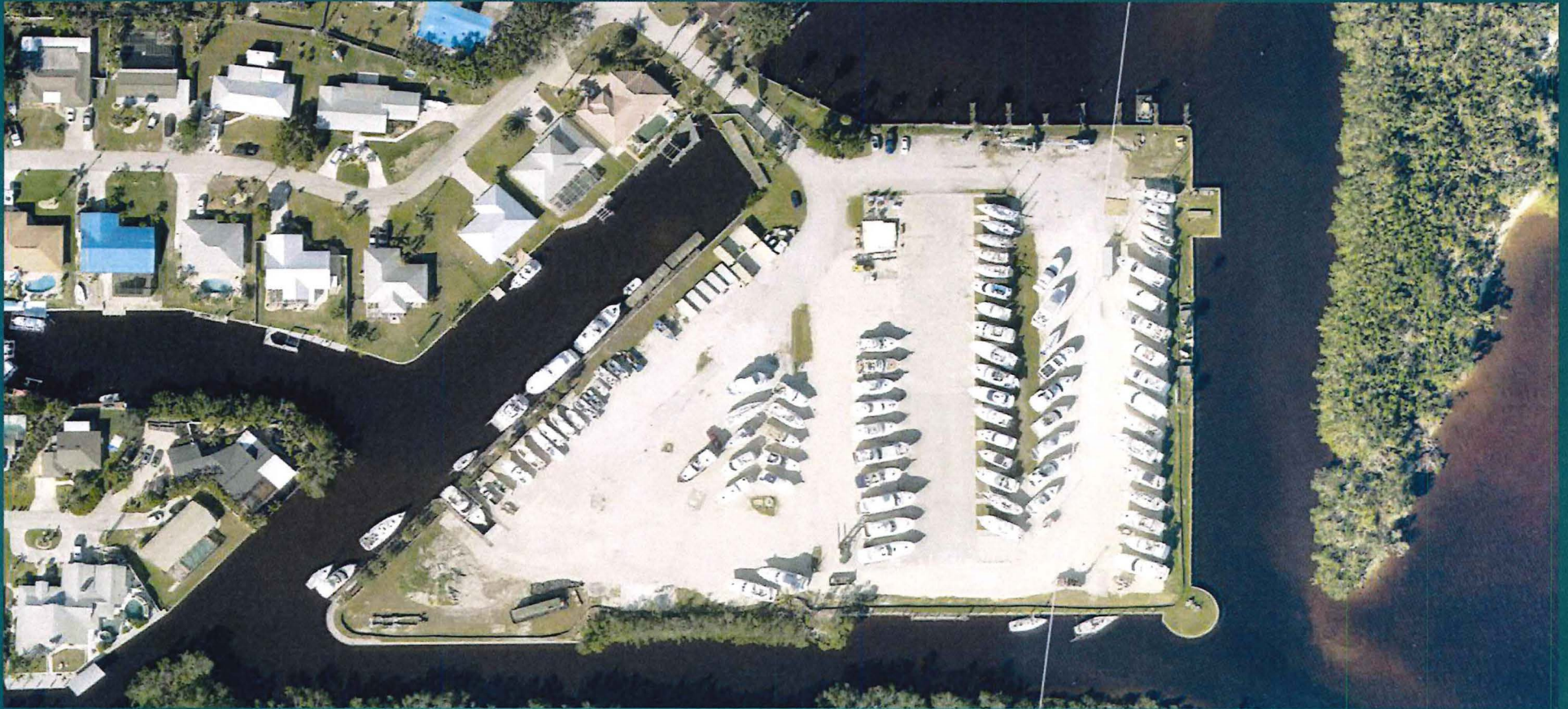
Existing Condition (During Previous Boat Triage Work)
