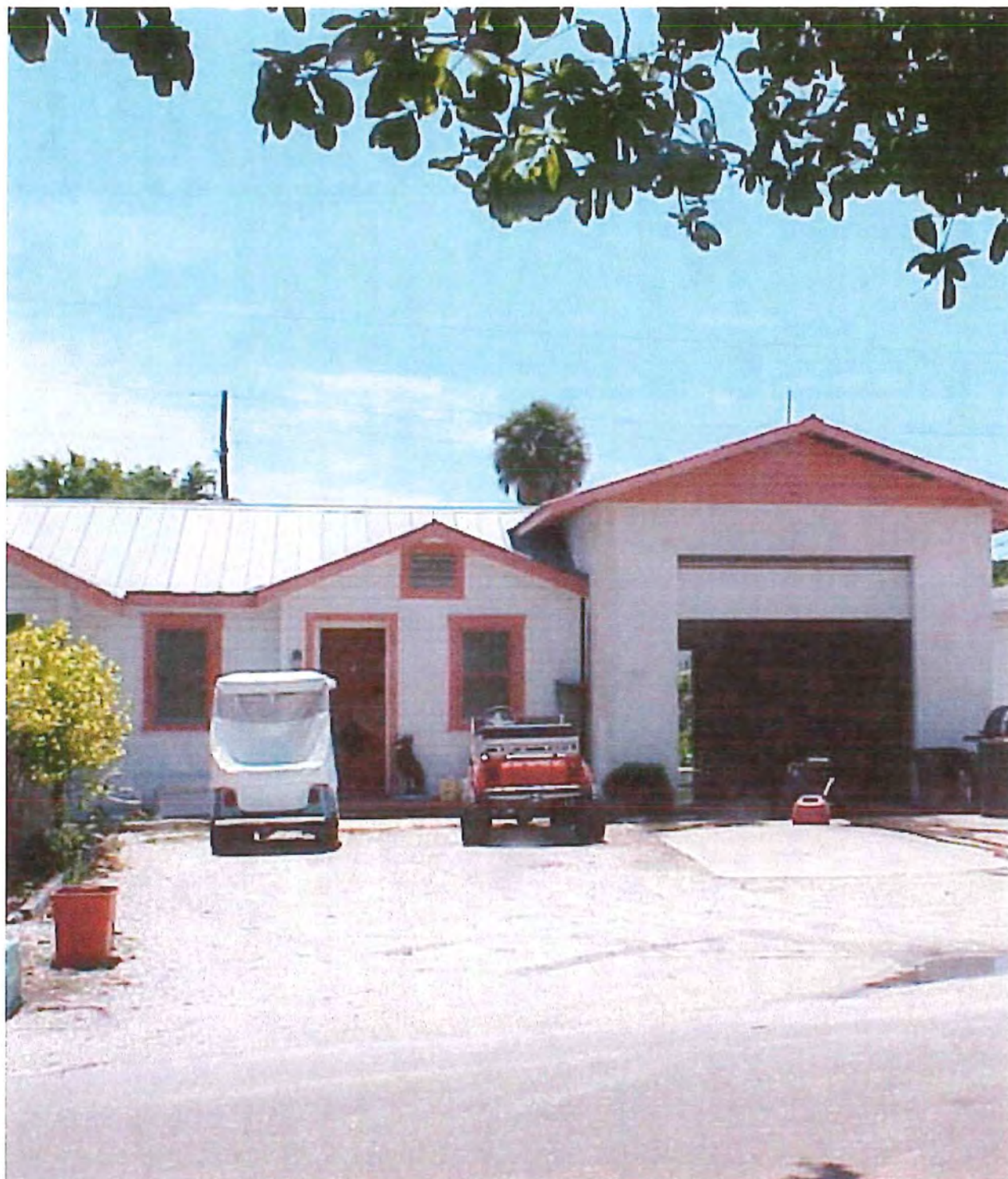
Front (east) elevation Palm Ave.
