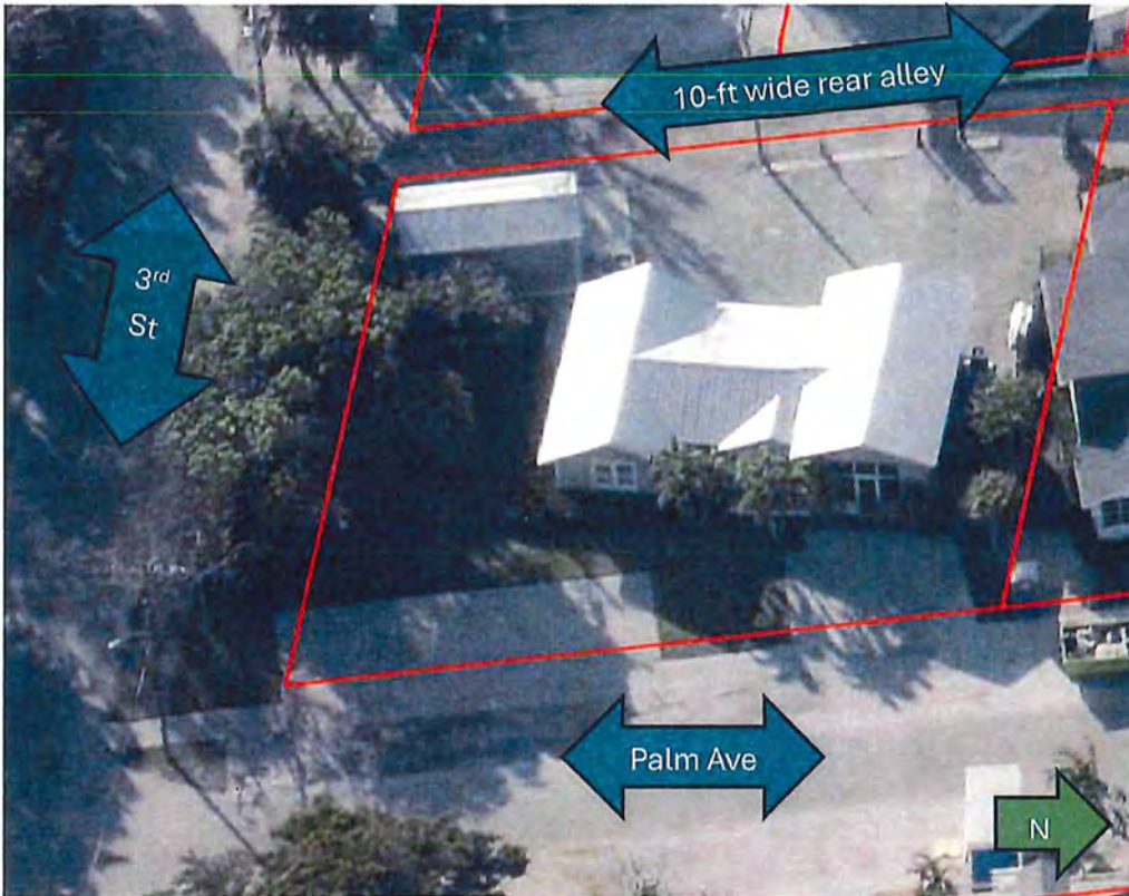
Aerial Front (east) elevation of the existing building
