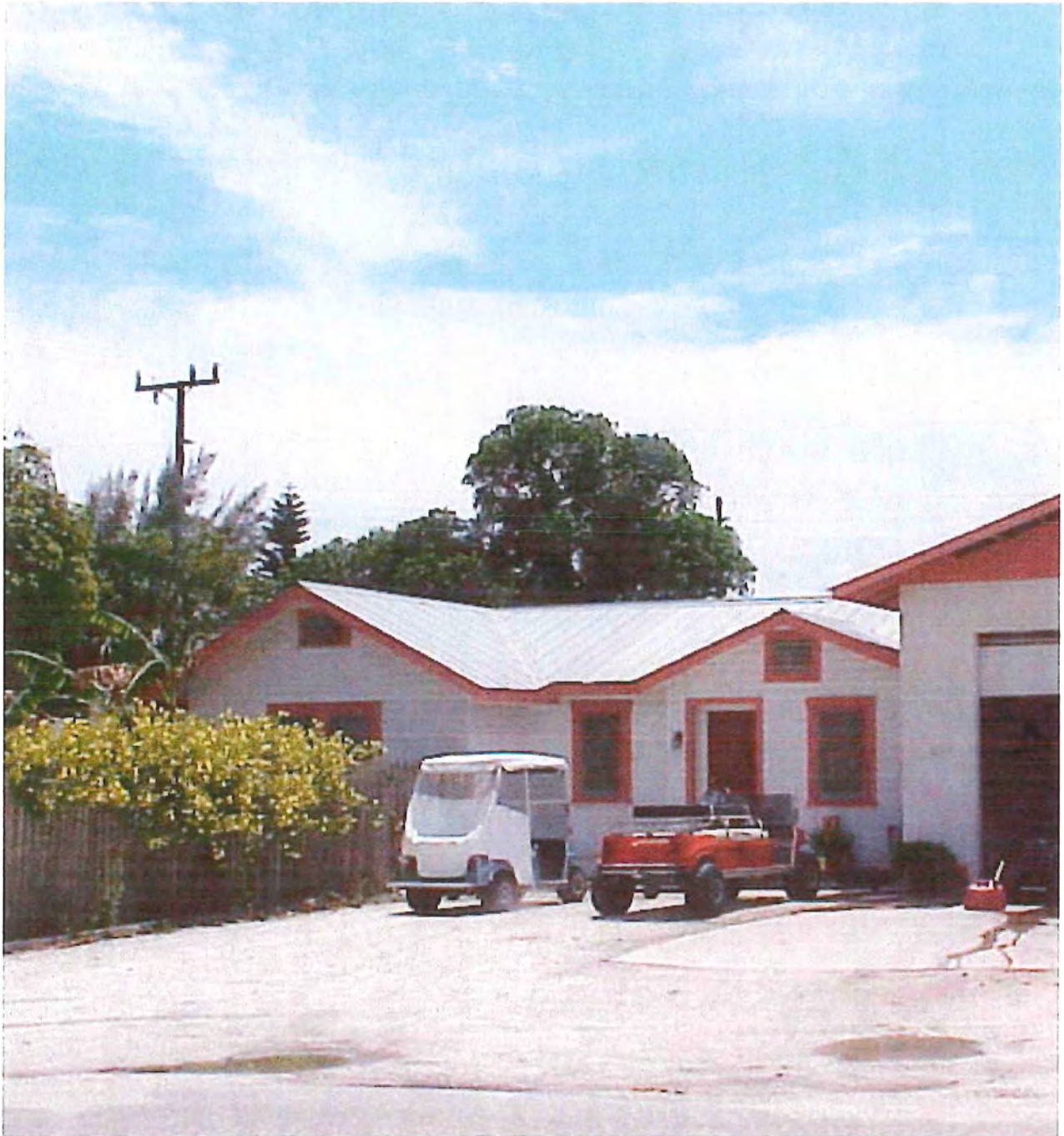
front (east) elevation Palm Ave.
