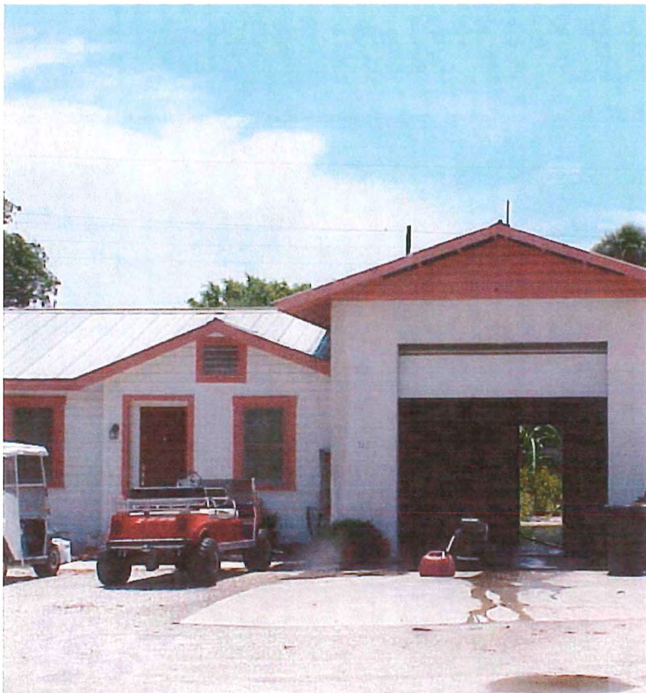
front (east) elevation Palm Ave.
