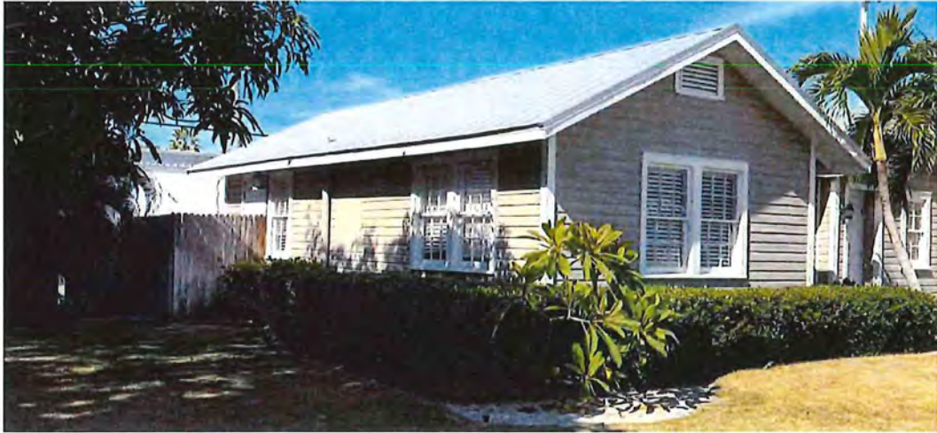
South (side) elevation of the south wing
