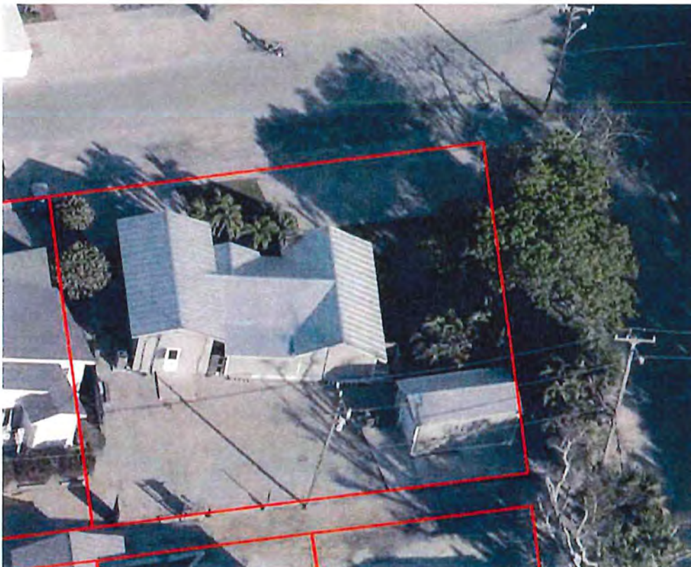
Aerial Rear (west) elevation of the existing building
