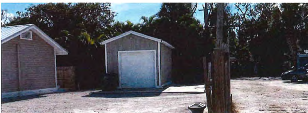
Shed at the rear by the alley will be demolished
