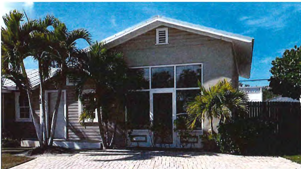
Close up detail of the north wing— the 1980s addition.
