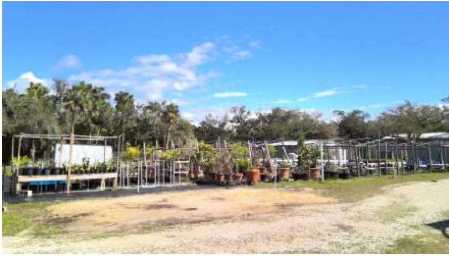
Building Front Photo
