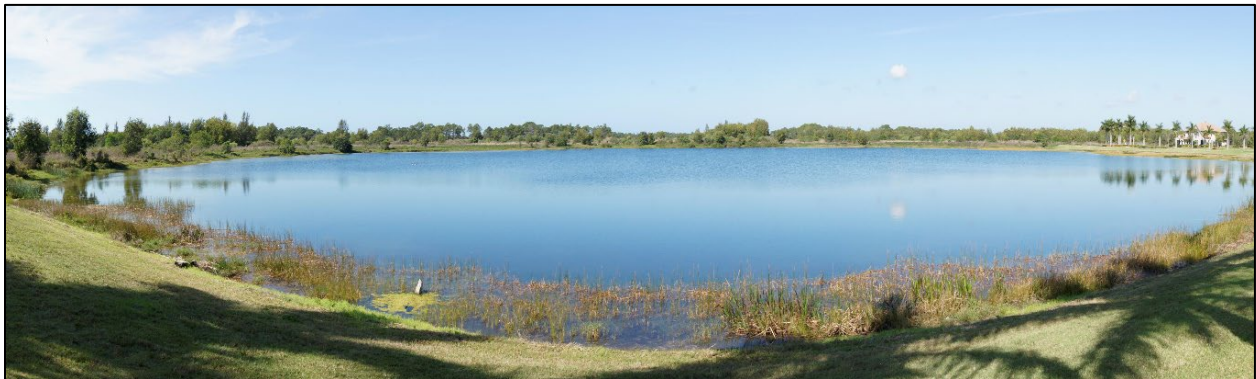
Figure 4. Typical Stormwater Management Lake
