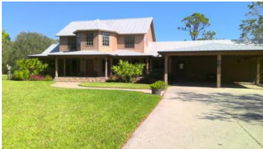
Building Front Photo
