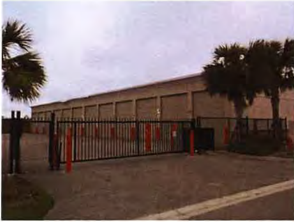
Building Front Photo
