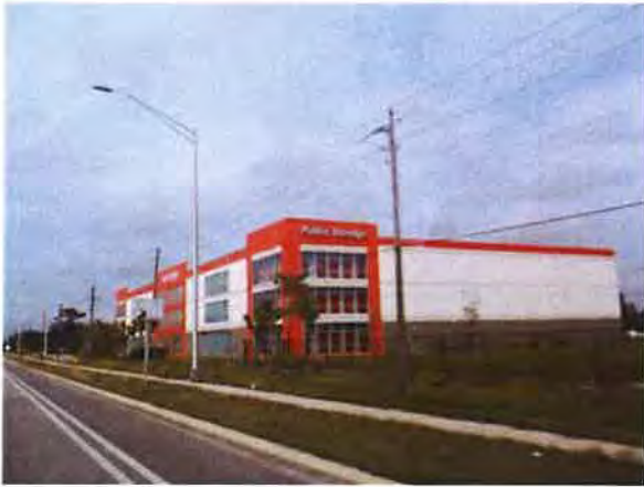
Building Front Photo
