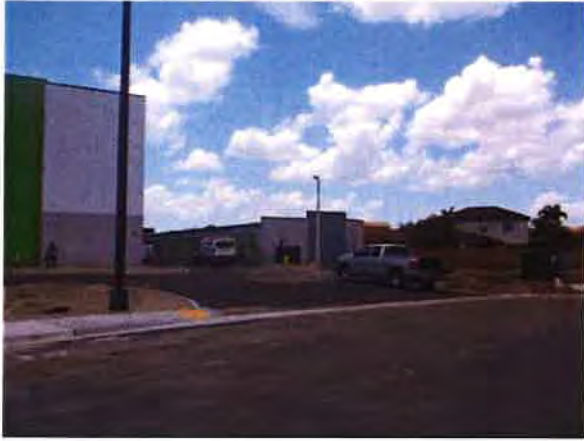
Building Front Photo
