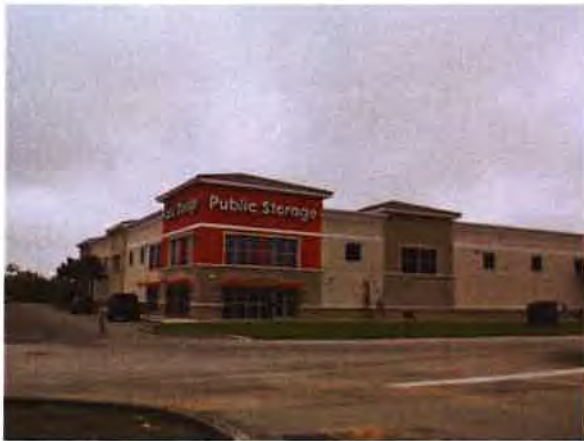
Building Front Photo
