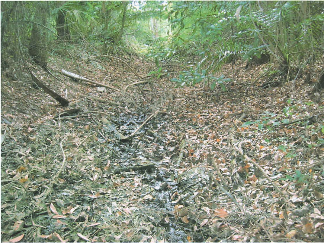
Ditch found along northern boundary.
