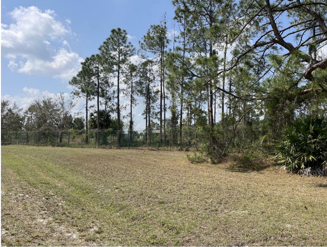
Drainage conveyance that runs the perimeter of property – View Southwest
