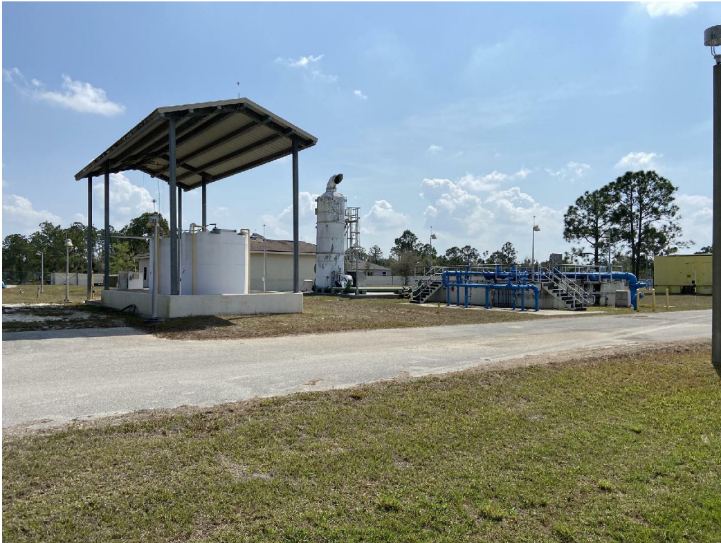
Currently facility on site – View East
