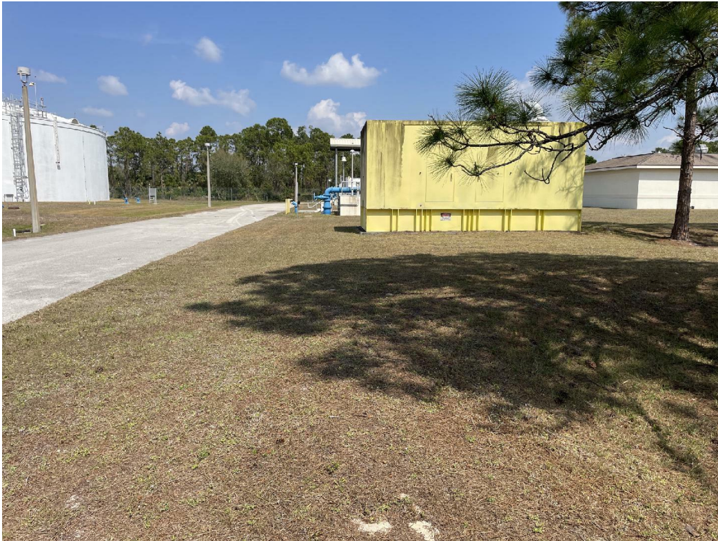
Representative site photo of current facility – View North
