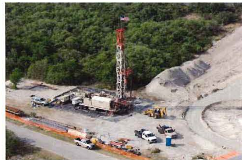
Well Drilling Operation
