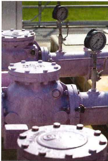
Reclaimed Water Piping
