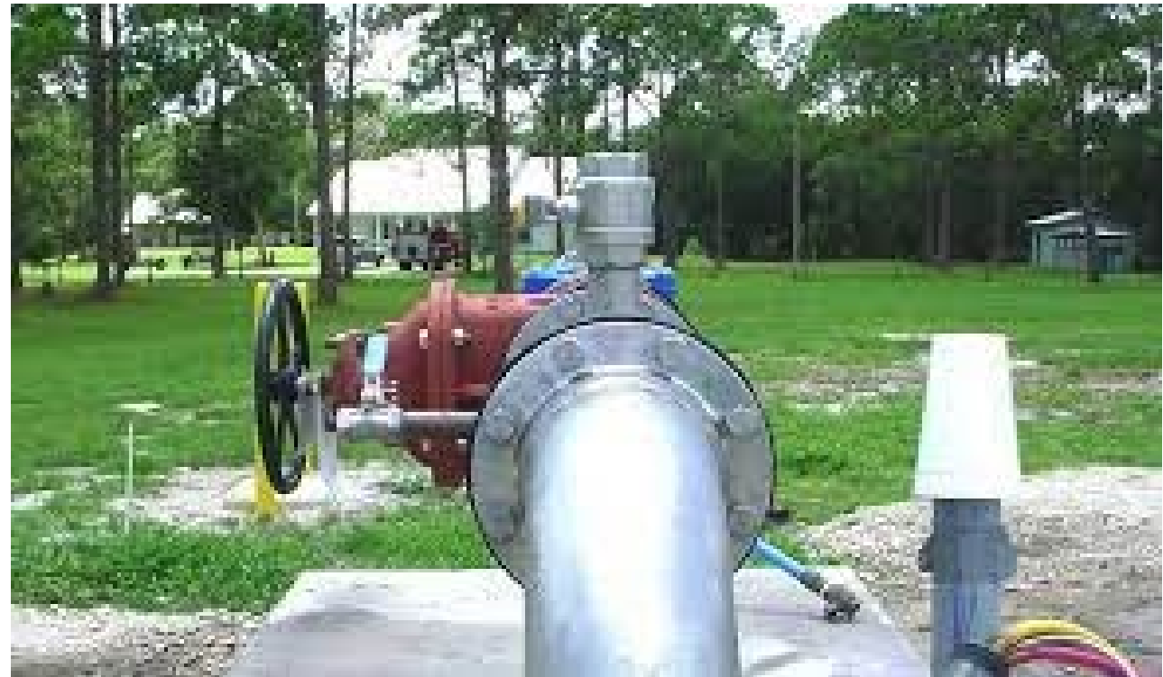
North Lee County RO Water Treatment Plant Expansion
