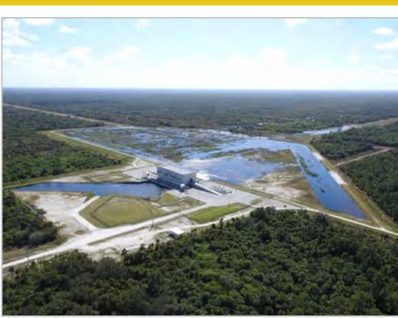
Merritt Pump Station
