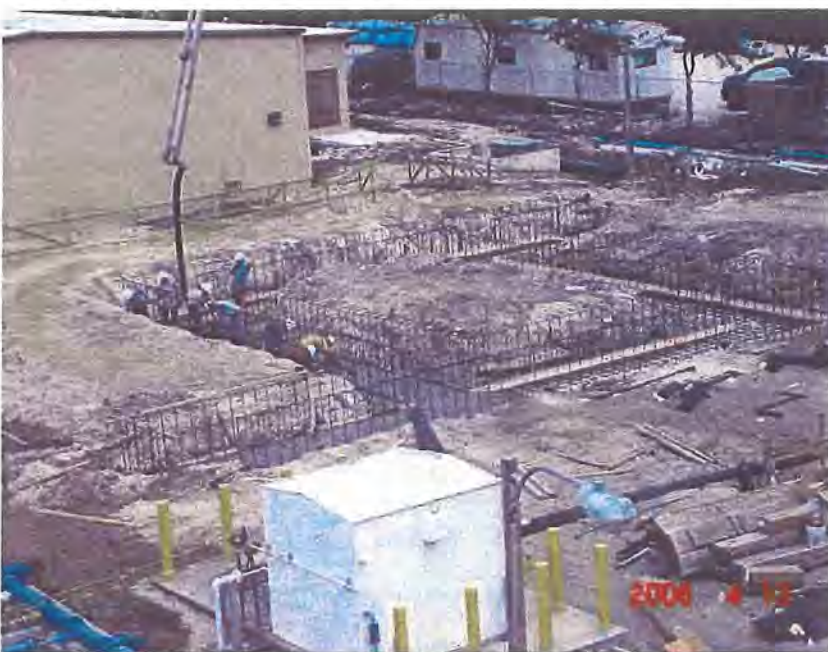
Construction of a 3 MGD reverse osmosis plant at the Pinewoods Water Treatment Plant. The existing plant is being expanded from 2.1 MGD to 2.3 MGD as part of the same contract.
