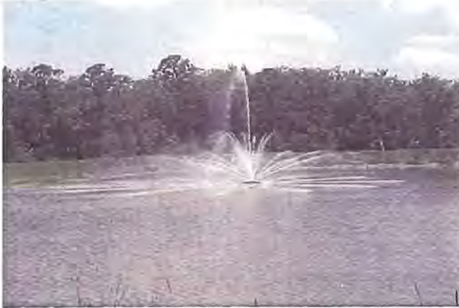
An aerator in a wet retention pond at River Hall to improve water quality.
