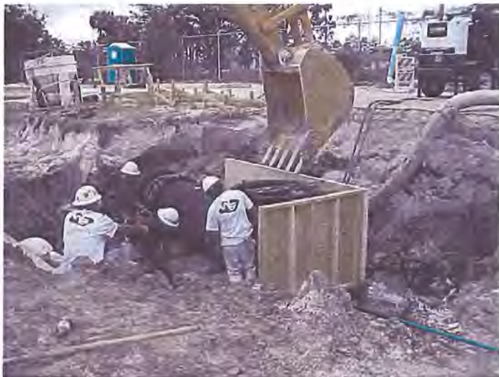
Installation of new piping at the Three Oaks STP in preparation for a contract to expand the plants capacity.
