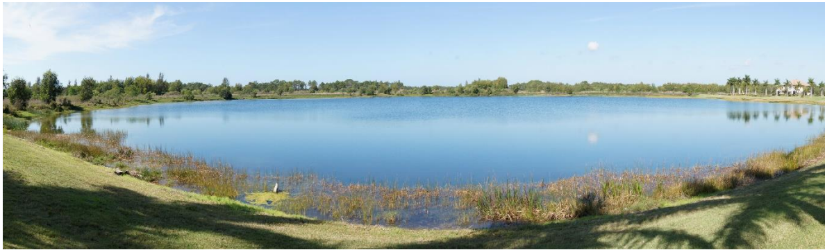
Figure 4. Typical Stormwater Management Lake
