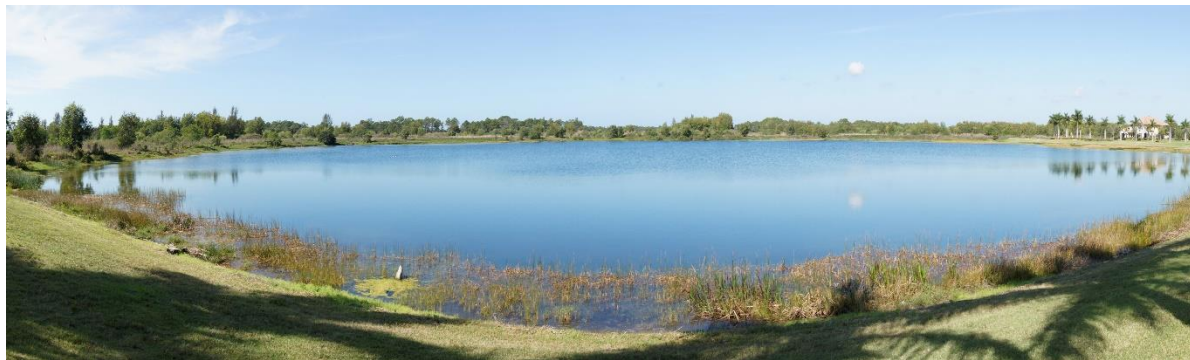
Figure 4. Typical Stormwater Management Lake
