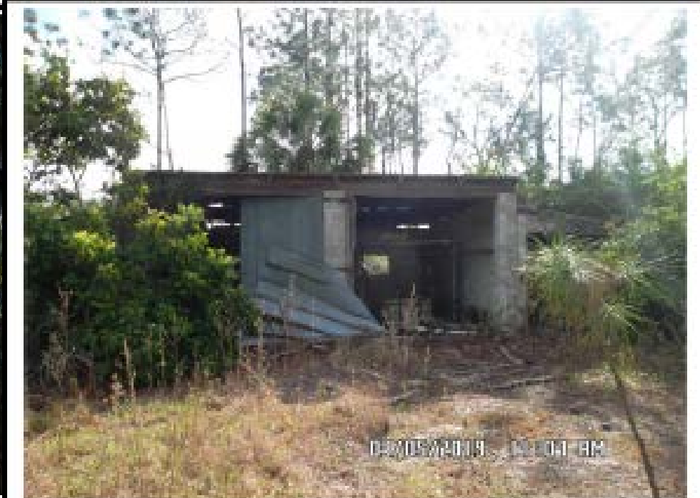
Photo 8 – View of the Small Shed
