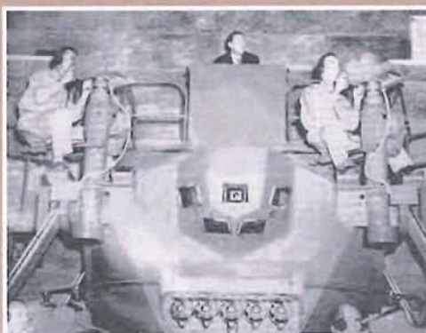
The Waller trainer used five motion picture projectors operating together and helped teach gunnery students the correct aim point for a moving target.
