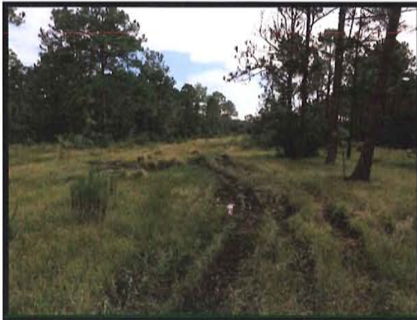
Upper Left Photograph: August 26, 2016 looking north along old farm road (vehicle ruts run along the eastern side of the elevated roadway (with the crest of the roadway to the left) at the reported Map 25 hydropattern connection. No culverts or defined flow-ways were observed at this location confirming that the historic farm road acts as sub-watershed boundary. Upper Right Photograph: August 26, 2016 looking along old farm road located to the east of Timber Creek that confirms SFWMD's sub-watershed boundary designation and isolates and separates the Timber Creek project from the balance of the DR/GR. No culverts or defined flow-ways were observed at any location along the old farm road.
