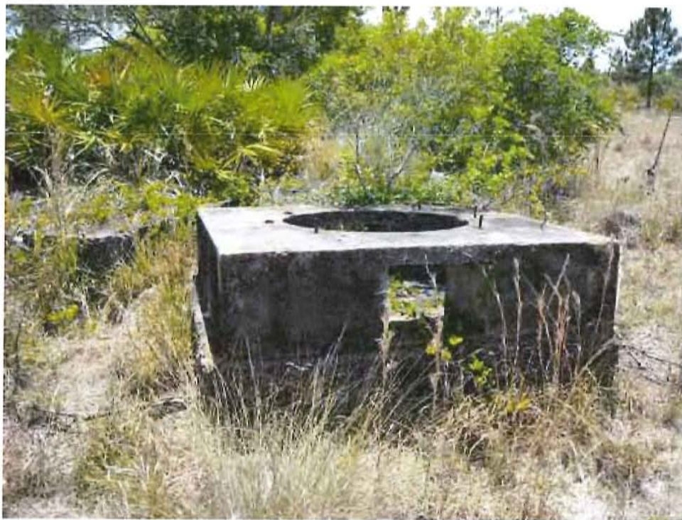
Figure 18. Concrete gun turret bases located adjacent to the limerock road within 8LL2552.
