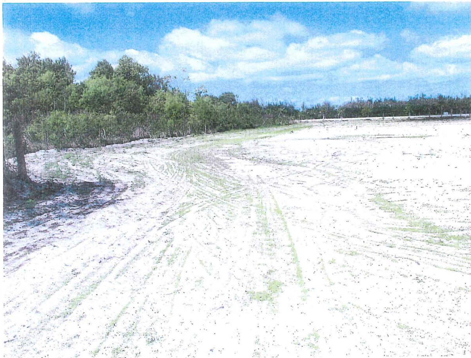
PHOTO #3: Collector swale has been excavated at the south end of the site. Seeded millet is becoming established.
