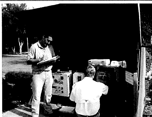
Water Conservation Audit – Irrigation Controller
