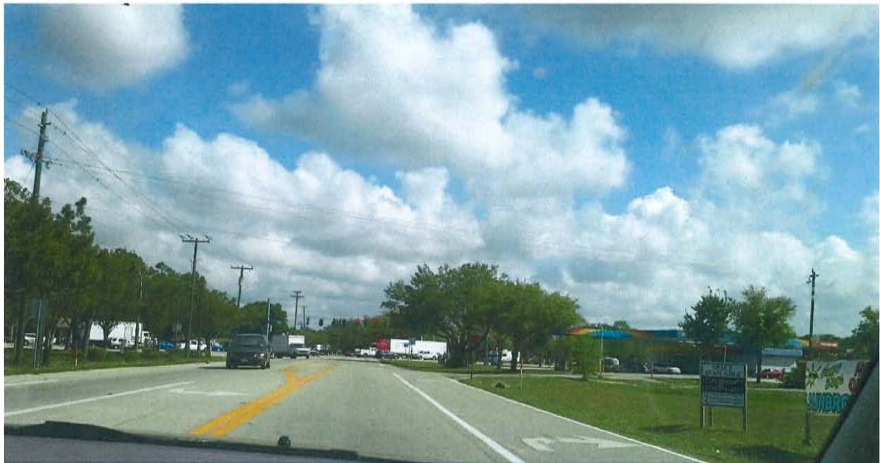
SR 80 looking eastbound at the Buckingham Road Intersection, March 2014. [Photo: J. Davis]
