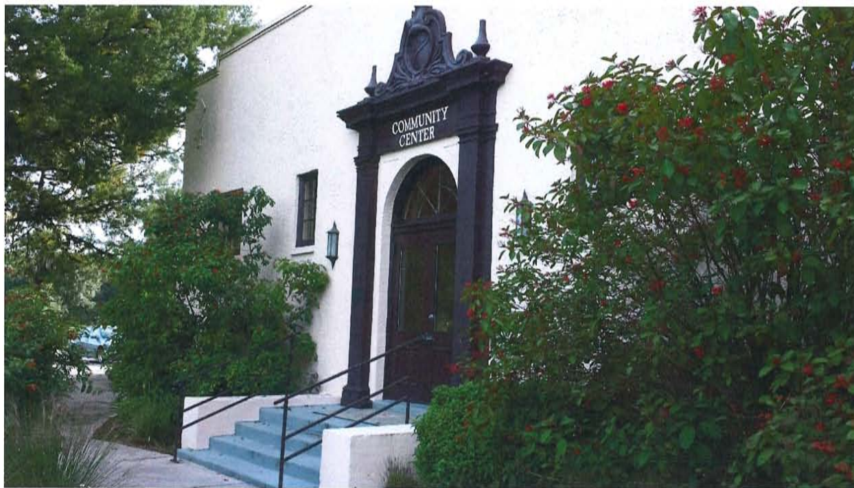
Olga Community Center, September 2014. [Photo: S Jenkins-Owen]
