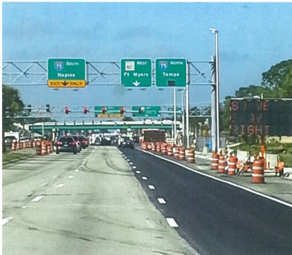
SR 80 at I-75 under construction, March 2014. [Photo: J. Davis]
