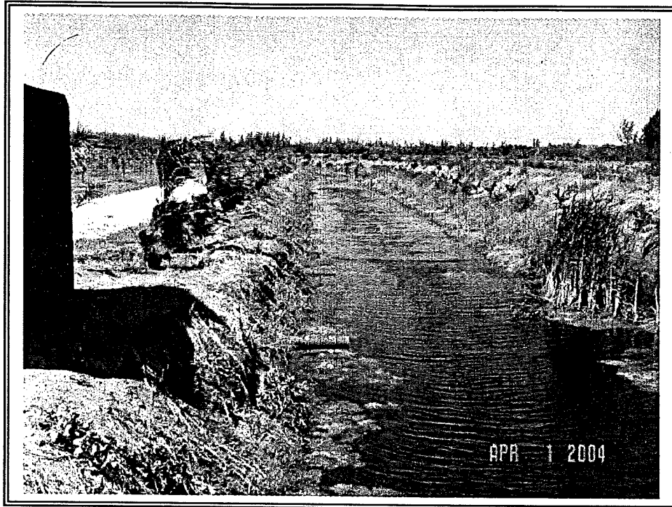
Photo No. 3: Photograph of canals within surface water management system.
