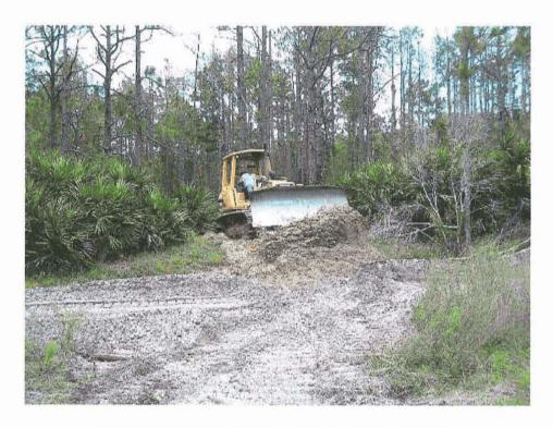
Breaching existing berm to restore sheet flow (2008)
