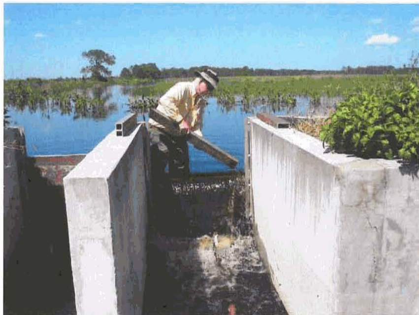
Releasing water to maintain appropriate water levels (2009)
