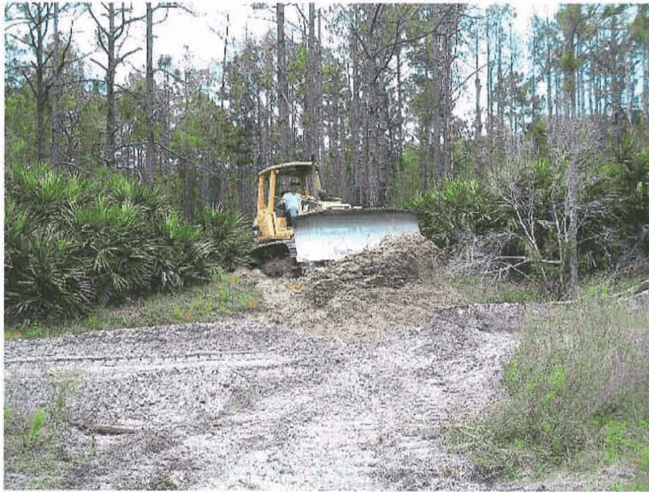
Breaching existing berm to restore sheet flow (2008)
