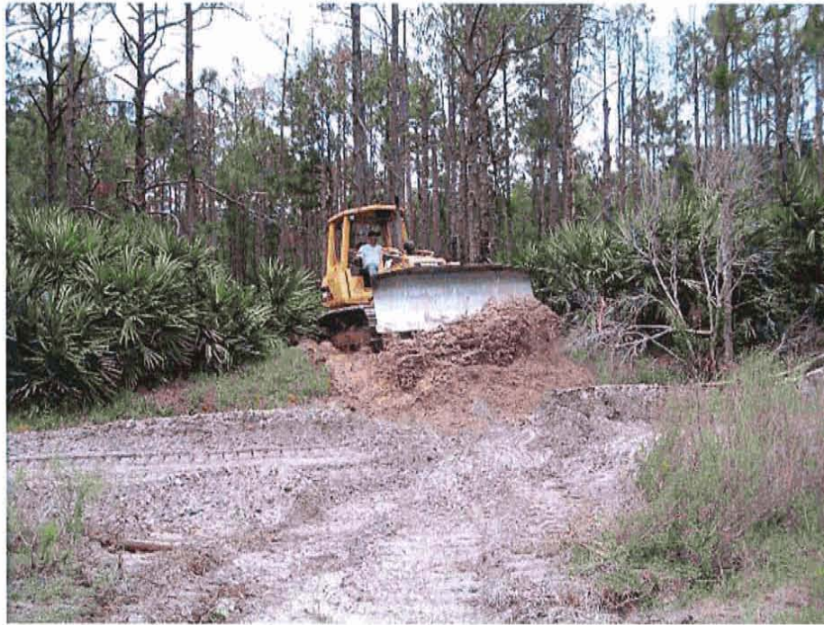
Breaching existing berm to restore sheet flow (2008)
