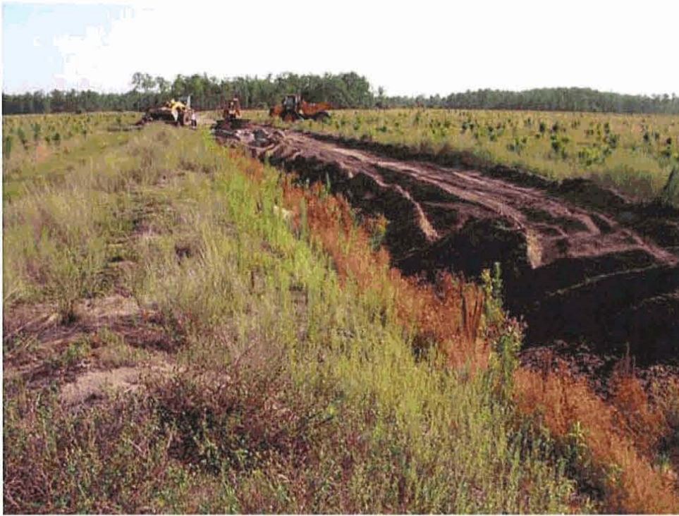
Backfilling agricultural ditches (2008)
