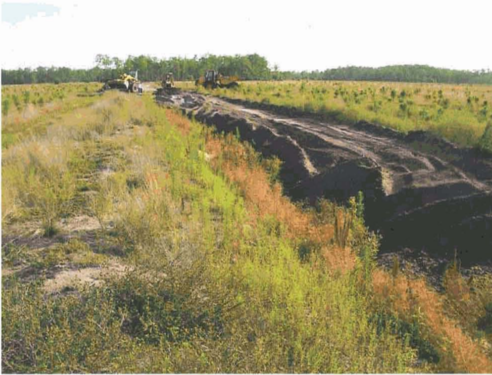
Backfilling agricultural ditches (2008)
