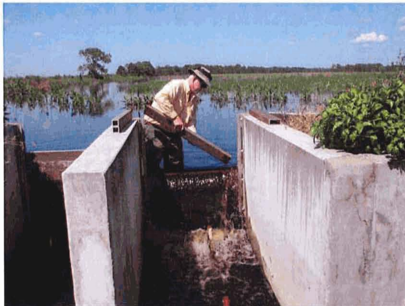
Releasing water to maintain appropriate water levels (2009)
