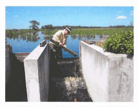
Releasing water to maintain appropriate water levels (2009)
