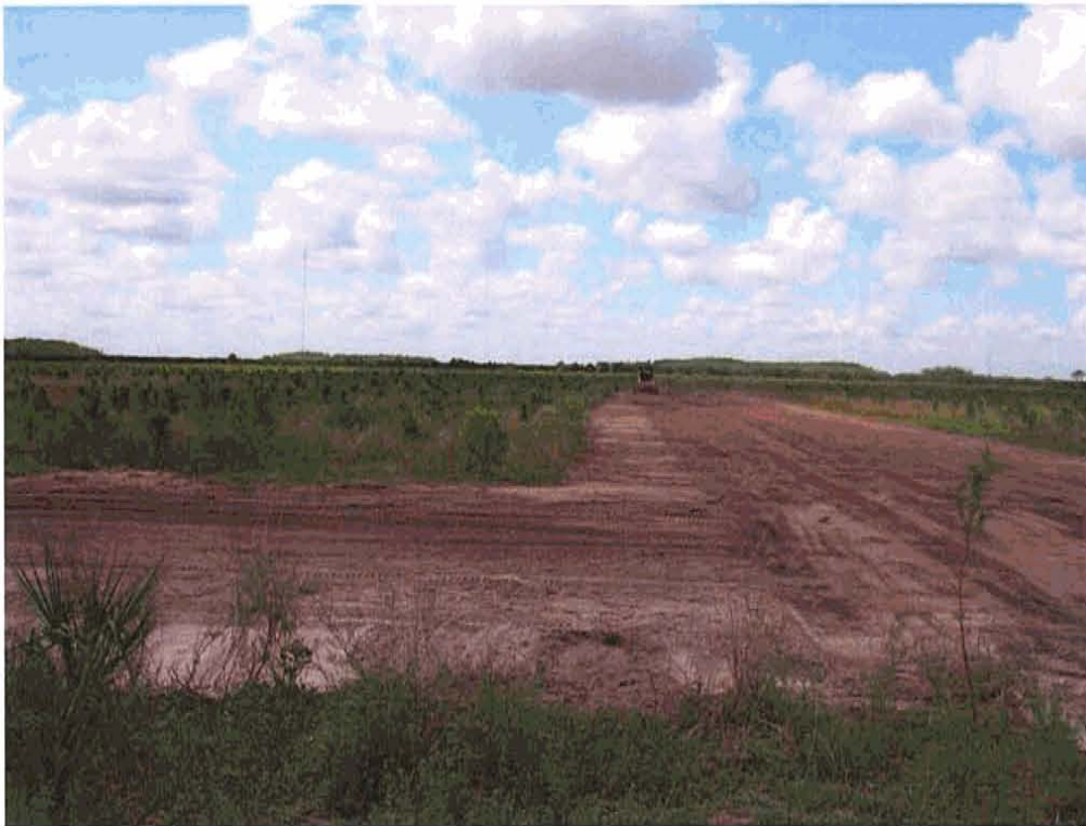
Backfilled and graded ditches to become hydric pine flatwoods (2008)
