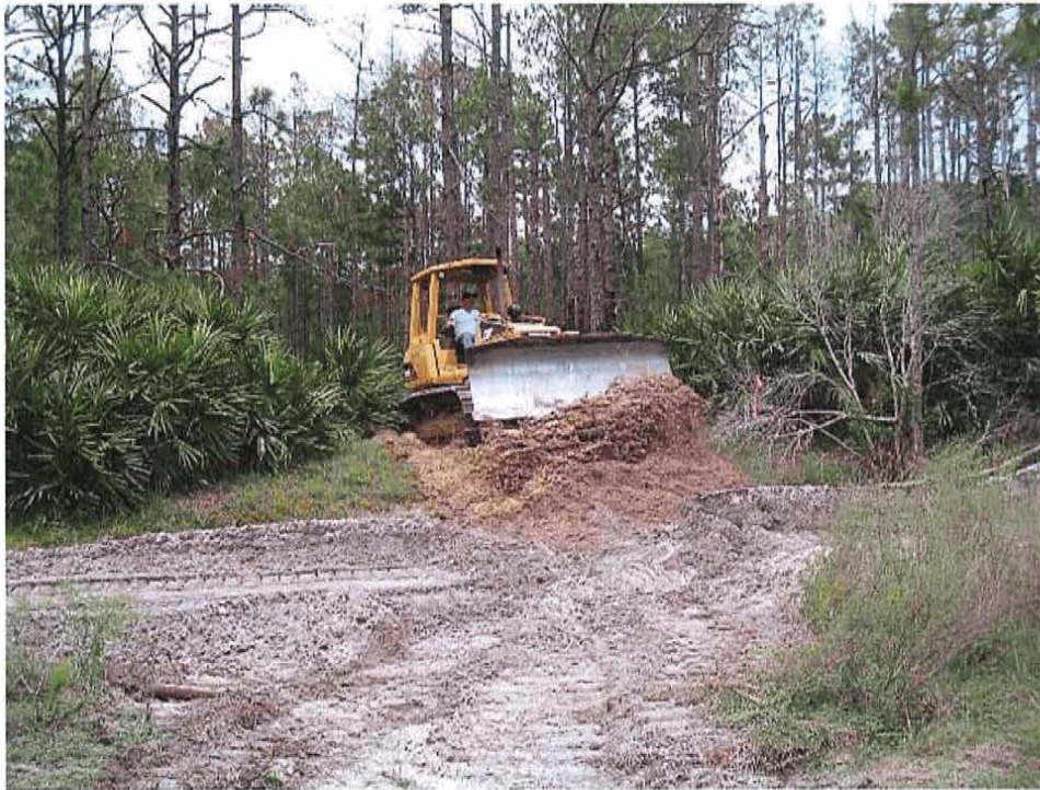
Breaching existing berm to restore sheet flow (2008)
