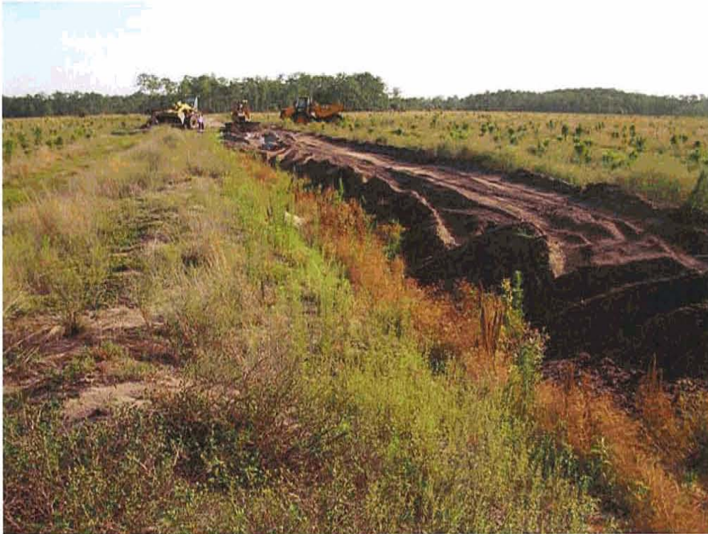
Backfilling agricultural ditches (2008)
