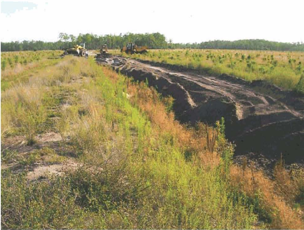
Backfilling agricultural ditches (2008)
