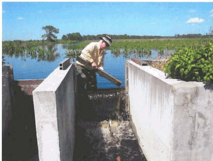
Releasing water to maintain appropriate water levels (2009)
