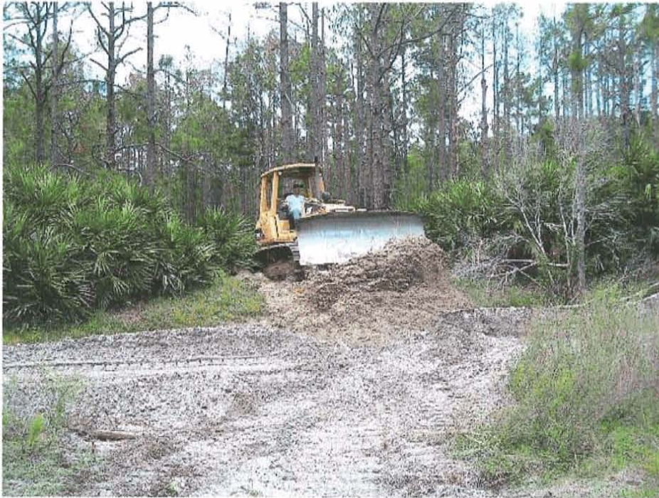
Breaching existing berm to restore sheet flow (2008)
