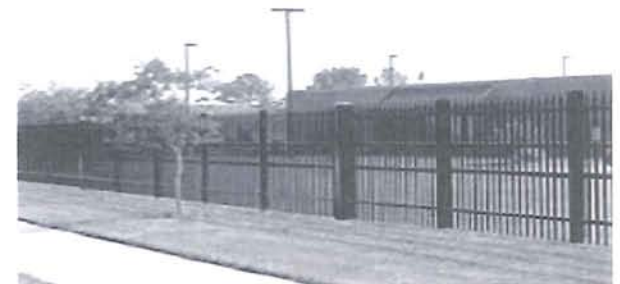
ALT. WROUGHT IRON PERIMETER FENCING ILLUSTRATION (Deviation 12)
