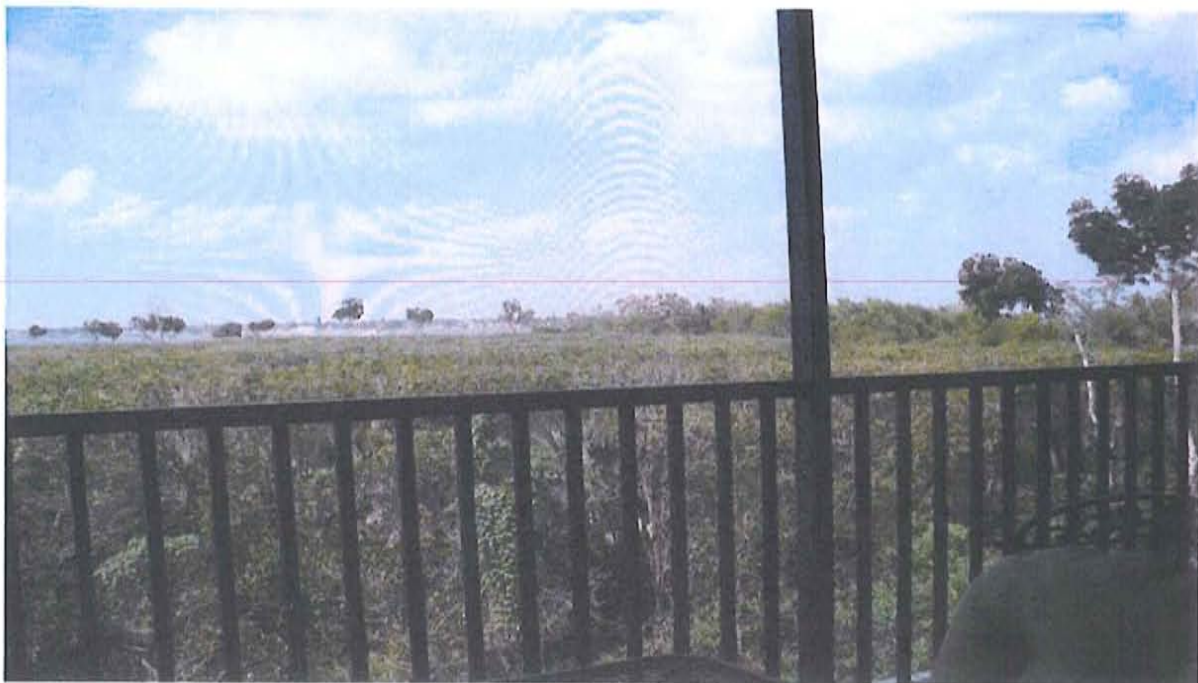
View looking upriver from the 1 st floor of the central building after recent trimming completed. 3/14
