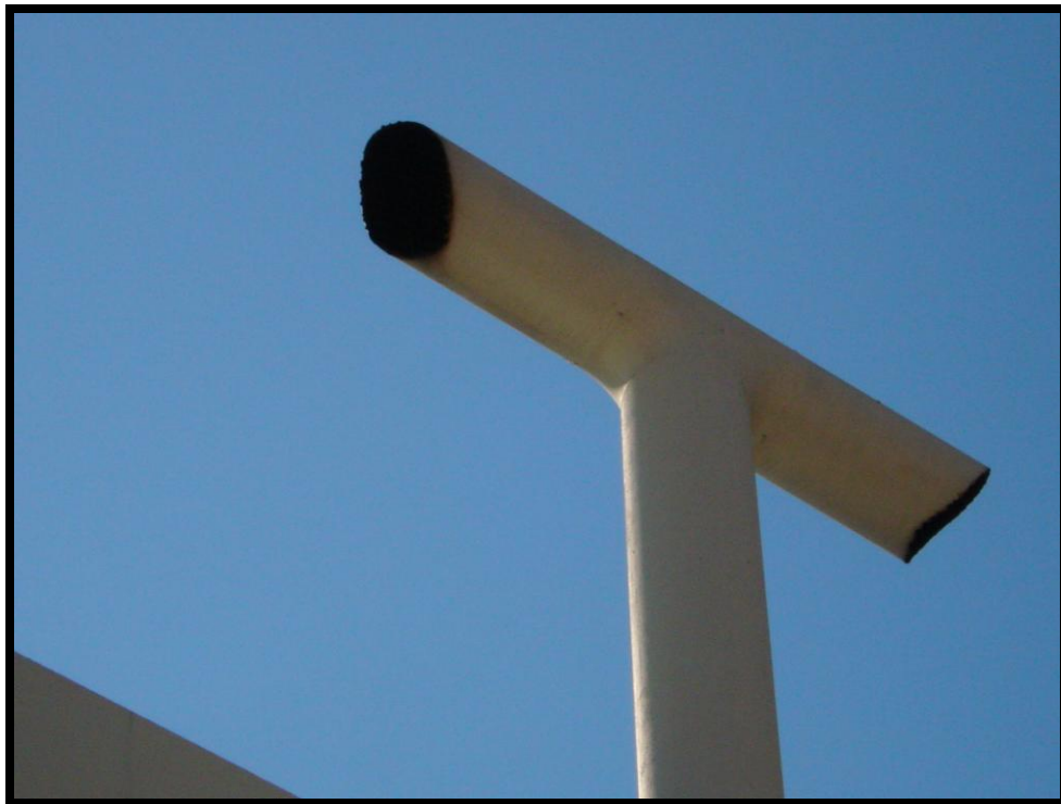
Typical exhaust vent with screen grating
