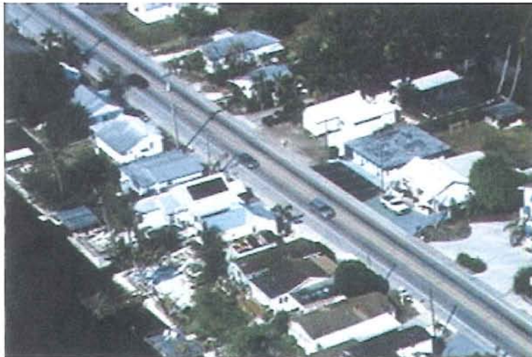
Matlacha historic district, bisected by Pine Island Road Photo courtesy of Mohsen Salehi and Bill Dubin
