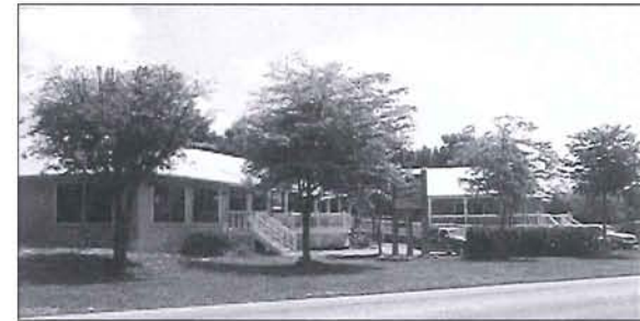
Island Exchange, Pine Island Center
