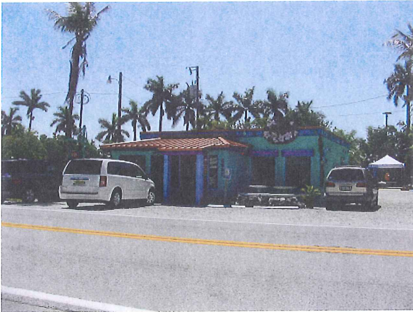
Front (north) elevation by Pine Island Rd.
