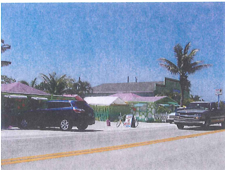
Buildings to the west side of the subject building
