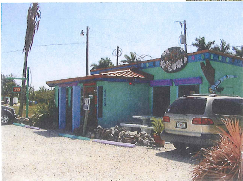
Front (north) elevation by Pine Island Rd.
