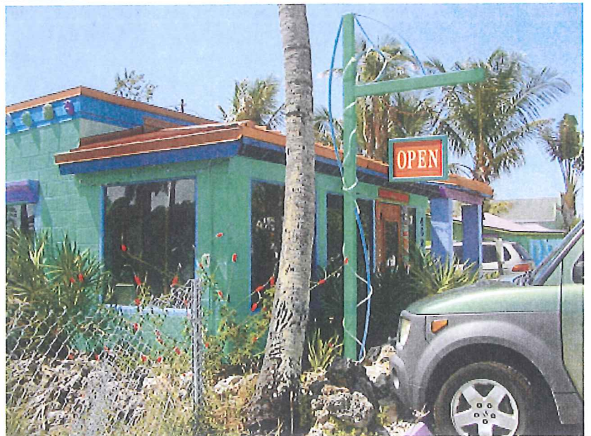
Front (north) elevation by Pine Island Rd.
