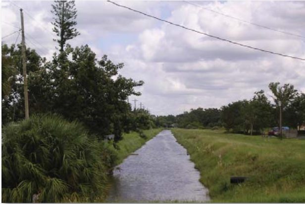
Lehigh Acres ECWCD Drainage Canals
